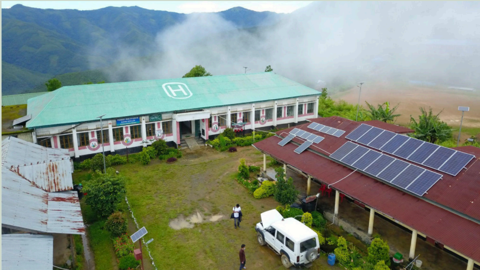
An aerial view of a Primary Health Centre in Manipur, India./SELCO Foundation
