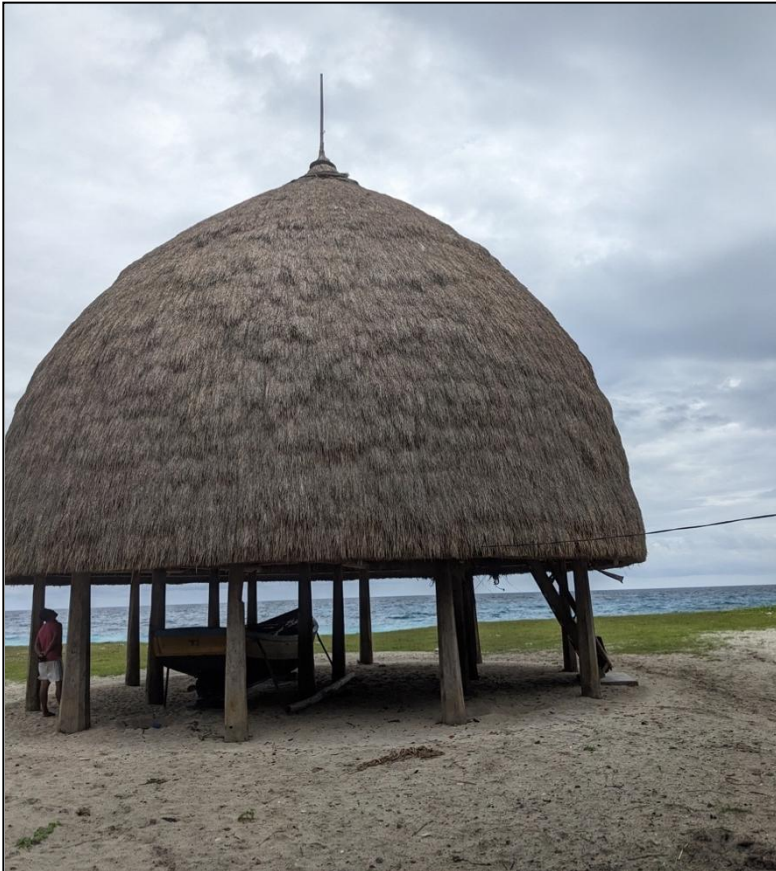
Figure 5: A Traditional House ( nyi hupul ) on the Island of Chowra; the Roof of the House Is Made of Grass Material Collected from the Community-owned Grasslands
