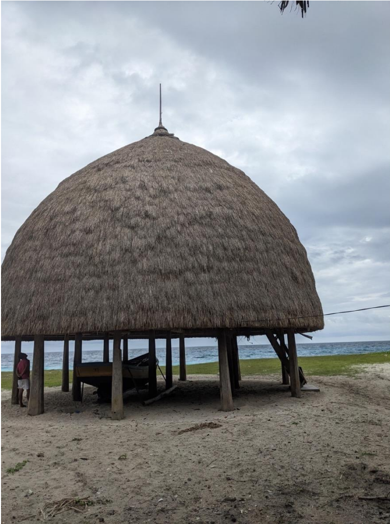
Figure 5: A Traditional House ( nyi hupul ) on the Island of Chowra; the Roof of the House Is Made of Grass Material Collected from the Community-owned Grasslands
